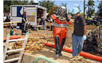
Greg West of Sea Engineering, who dived through 600 feet of sewer pipe to examine it for leaks, calls his job "adventurous" and "fun."
